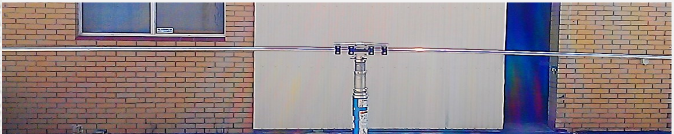
Rear view showing the method of attachment to an optional round 50mm vertical masthead.
